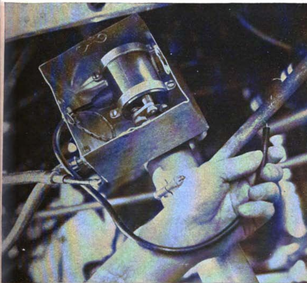
Figure 77. Checking booster-coil spark strength.
