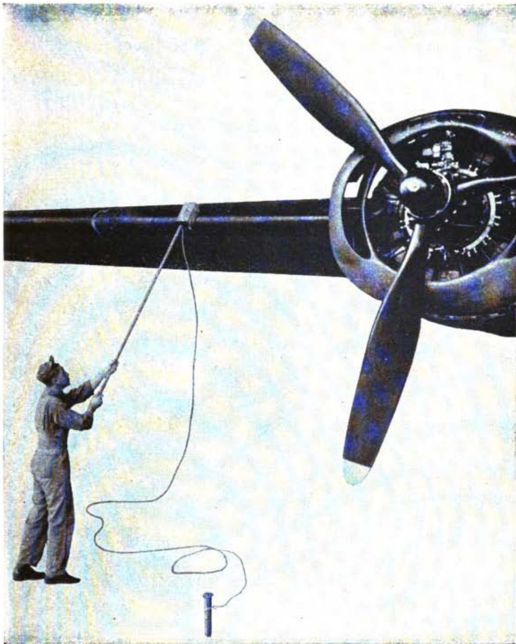
Figure 45. Grounding de-icer shoes.
