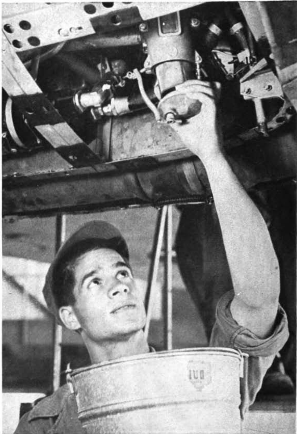
Figure 59. Removing main-line strainer for cleaning.
