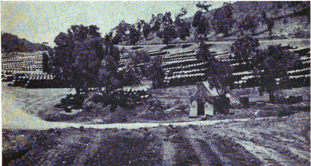
Figure 17. Petroleum storage area in the Southwest Pacific. Hillside site provides good natural drainage. No dispersion is practiced here.
