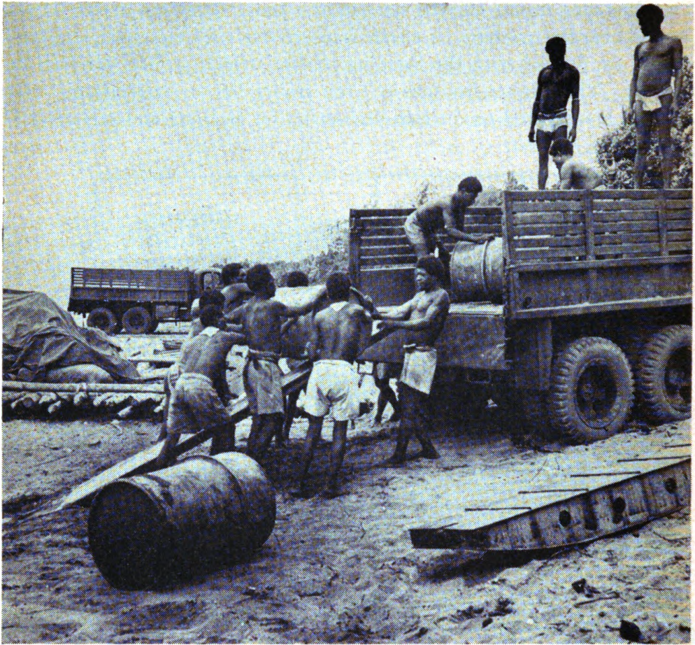
Figure 7. Skids used by native laborers in loading 55-gallon drums into truck.
