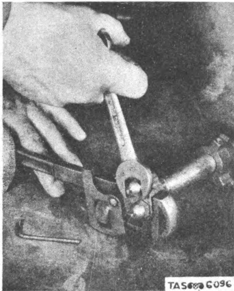
Fig. 96. Removing Nozzle.
