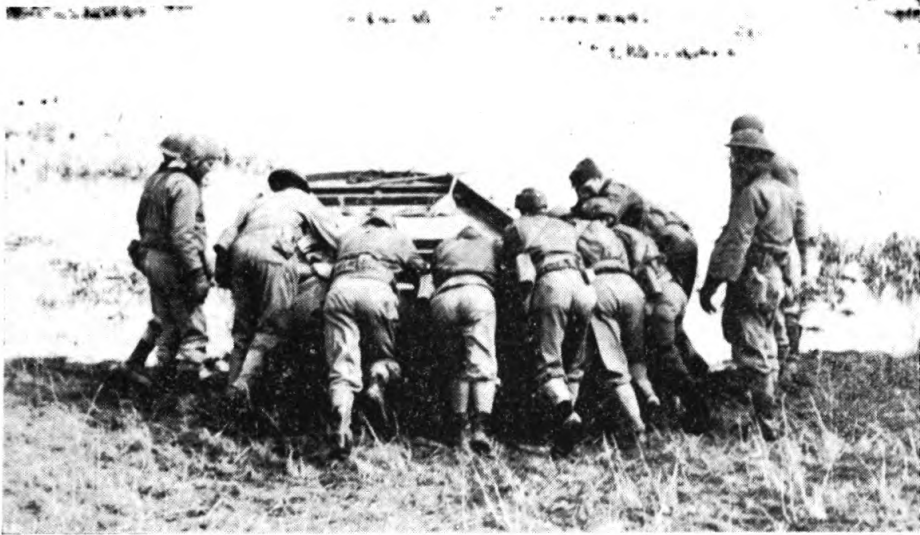
Figure 21. Launching Ponton.
