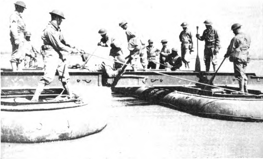
Figure 25. Installing connecting pins.
