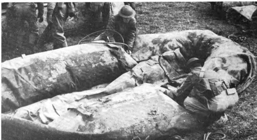
Figure 20. Inflating Pneumatic Float.
