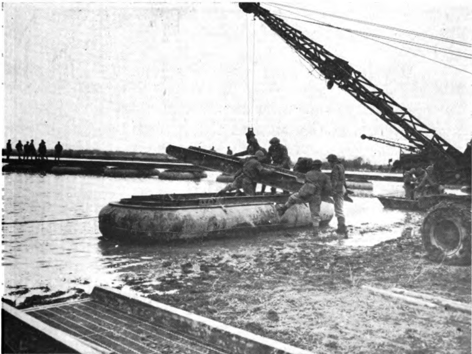
Figure 22. Placing treadways in assembling a ponton section.
