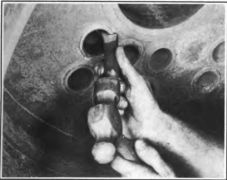
FIG. 62 Beading New Tube End
