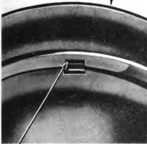
INSPECTION OPENING WITH THE COVER REMOVED 1—DRUM INSPECTION HOLE
